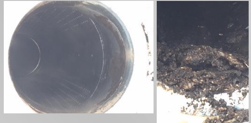
BC distribution header after chemical cleaning
