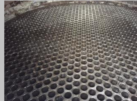
BC tube sheet after hydro-blast
