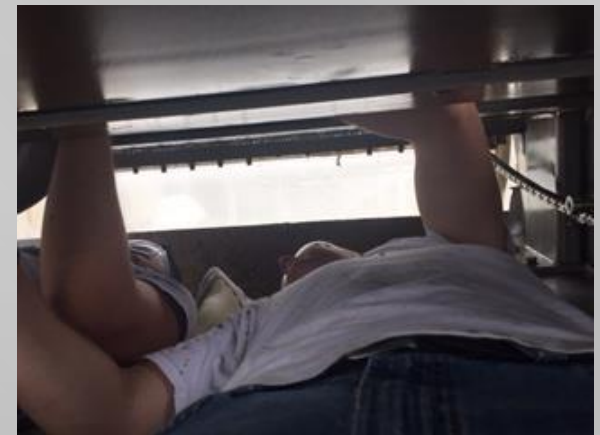
Hard at work WTO's repairing F. P leak
